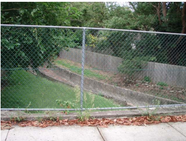
Plate 3 Macquarie St. Looking Upstream at Low Lying Residential Allotments Northern Side of SW Channel
