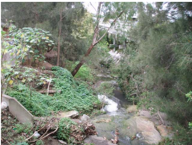
Plate 11 Improved Channel Looking Downstream from Gibbes St. Bridge
