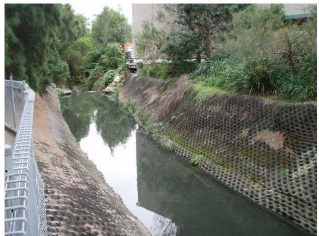
Plate 6 Looking Downstream at Rock Weir on Downstream Side Retirement Village
