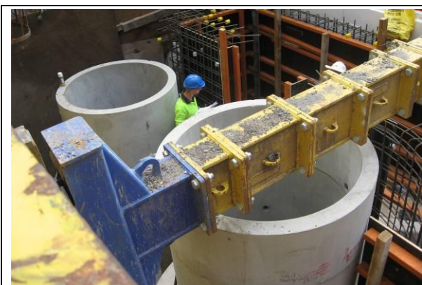
CDS units being installed
