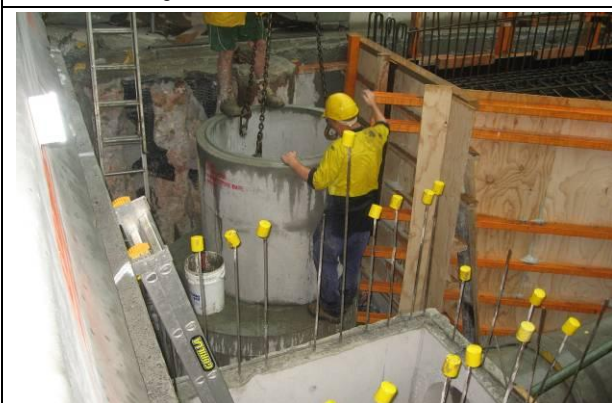
CDS unit being installed
