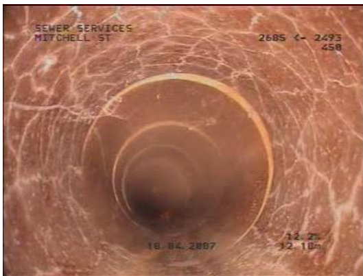
Crocodile Cracking
