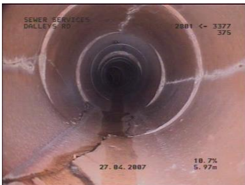
Quadrant Cracking
