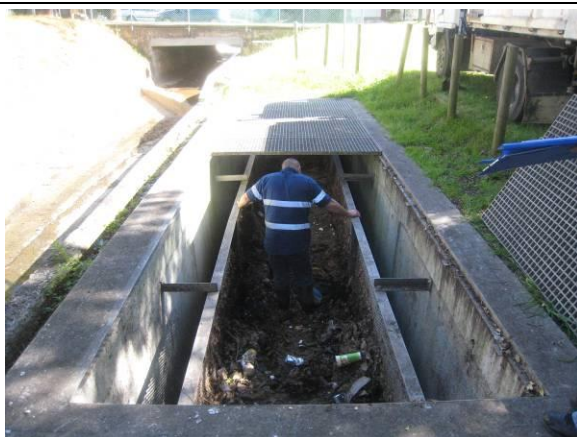
Baramy at Crick St being cleaned.
