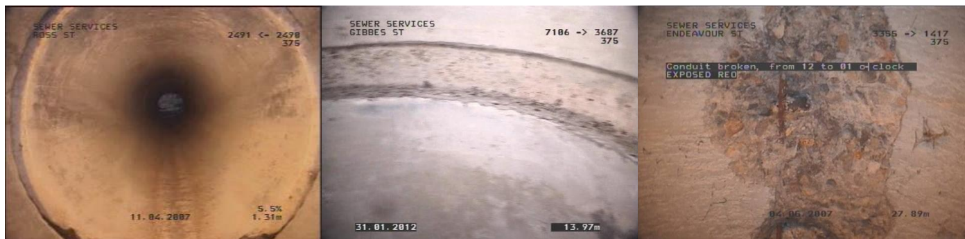
Medium displaced joint
