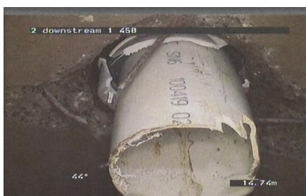
Minor object intrusion
