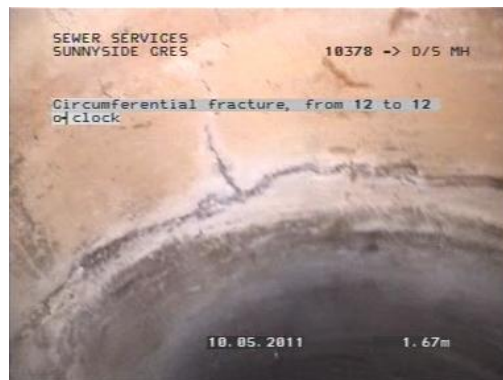
Circumferential Cracking
