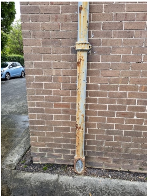
Figure 40 original rainwater goods of the main 1932 school building.
