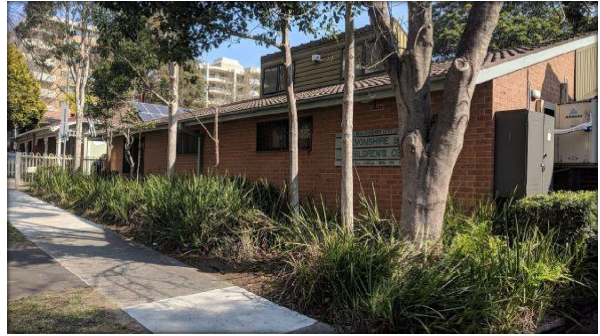
34 and 40 Devonshire Street from Devonshire Street frontage
