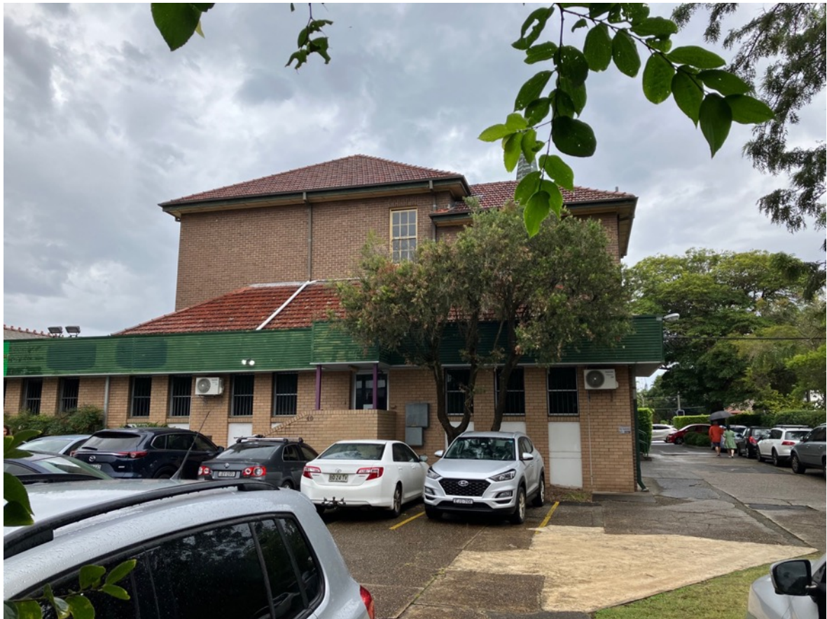
Figure 35 northern elevation of the 1932 main school building, which appears to have a single storey accretion that links this to the single storey classroom building (ridge capping seen in the distance).
