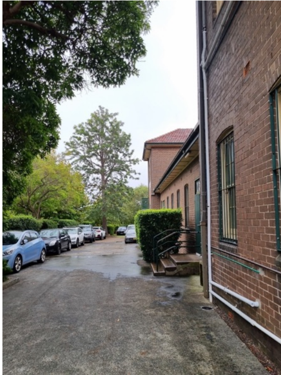
Figure 38 western elevation of the 1932 main school building fronting Willoughby Road
