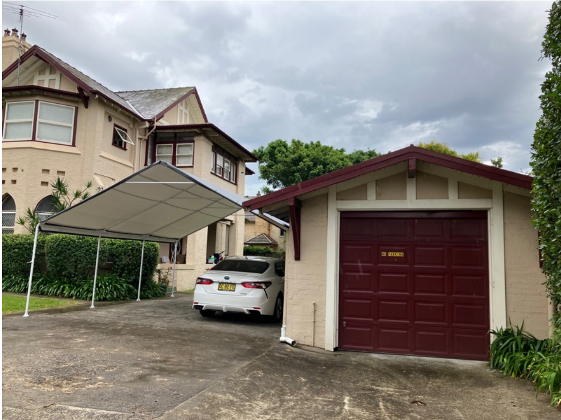
Figure 29 The 1917 Garage, the second element in the sequence of construction after the church.
