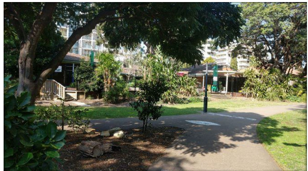
40 Devonshire Street from Tingha Street
