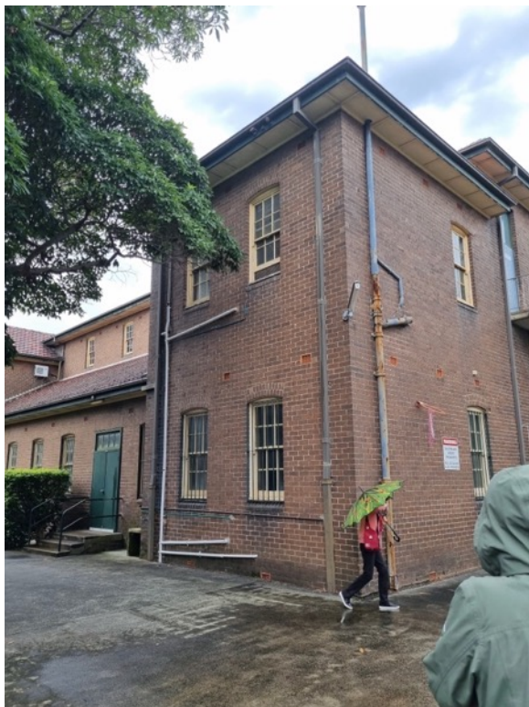
Figure 31 south-western corner of the 1932 main school building, hall and annex
