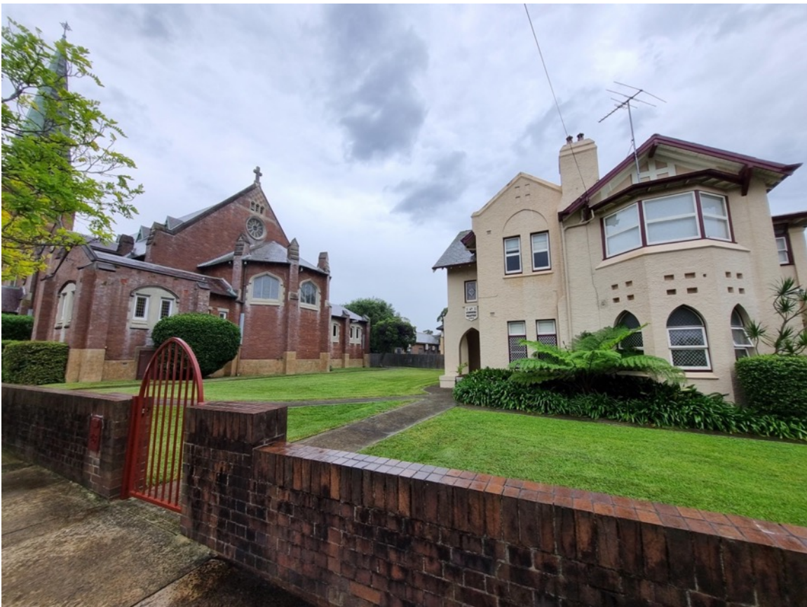
Figure 30 View of the rectory in the context of the adjoining church from Donnelly Road.
