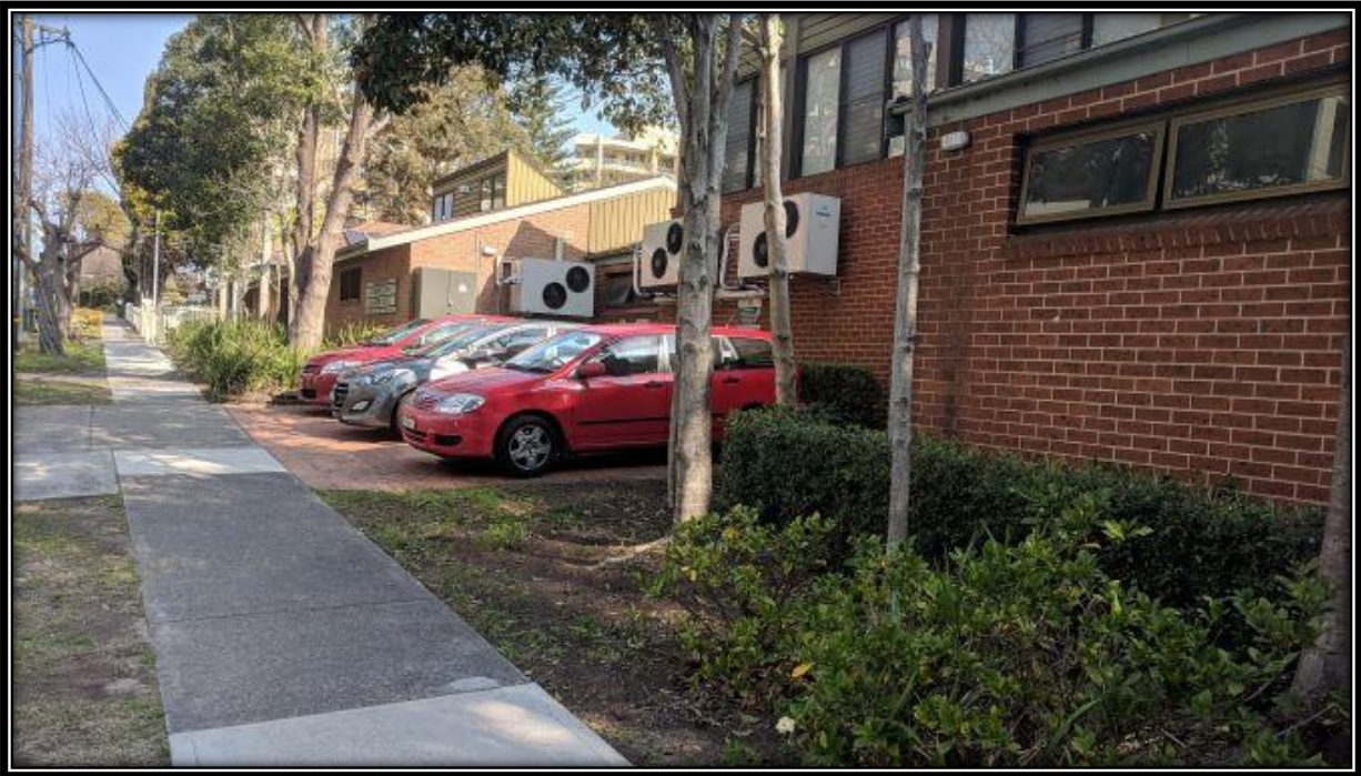
Photo 6 – 40 Devonshire Street from Devonshire Street frontage
