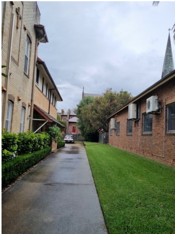
Figure 44 eastern elevation of single storey 1936 building and its relationship to the adjacent 1935 Sisters of St Josephs building.
