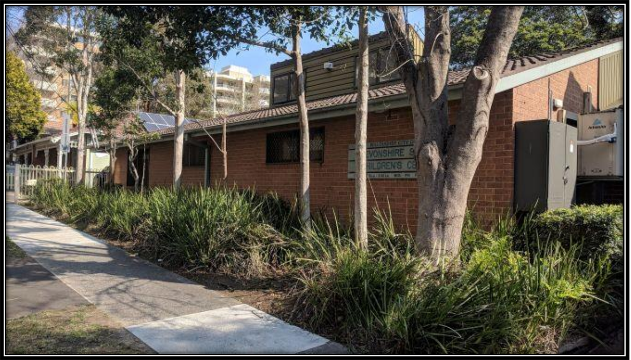
Photo 7 – 34 and 40 Devonshire Street from Devonshire Street frontage
