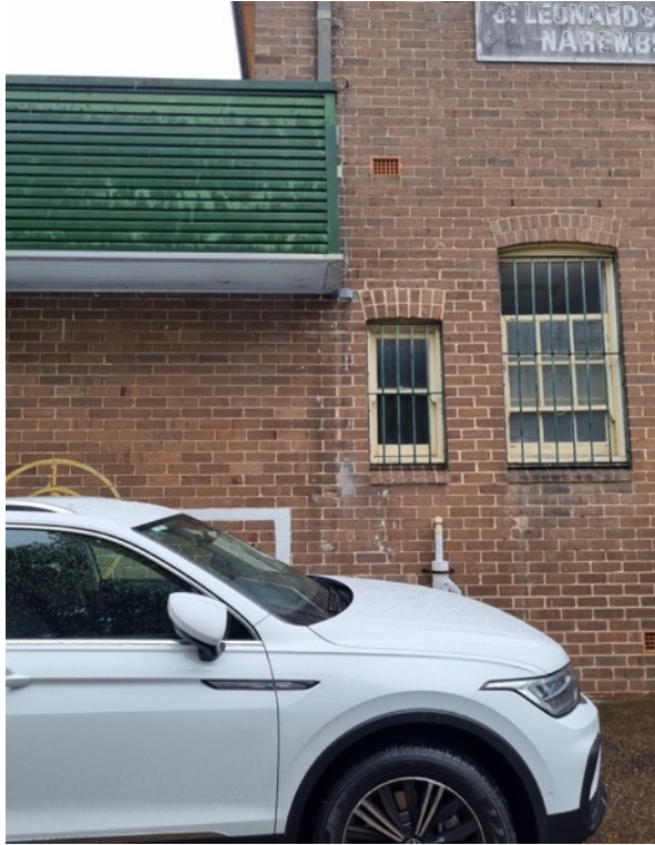
Figure 33 accretion at the northern end of the 1932 main school building.
