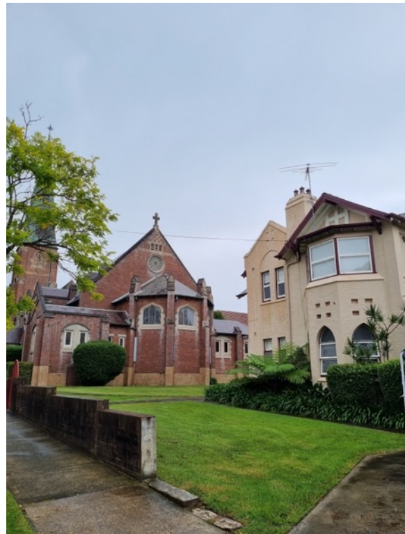
Figure 27 Grounds to the front of the presbytery
