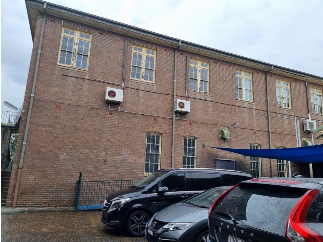
Figure 36 eastern elevation of the 1932 two-storey main school building (hall and annex).
