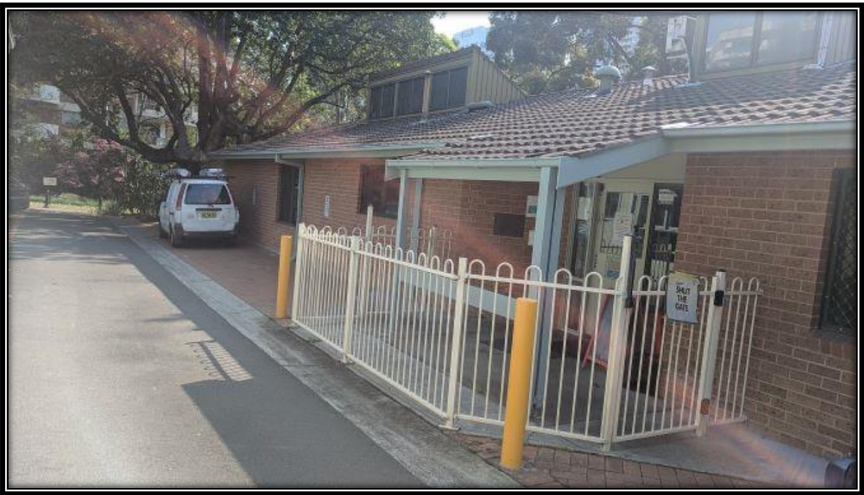
Photo 10 – 40 Devonshire Street southern elevation
