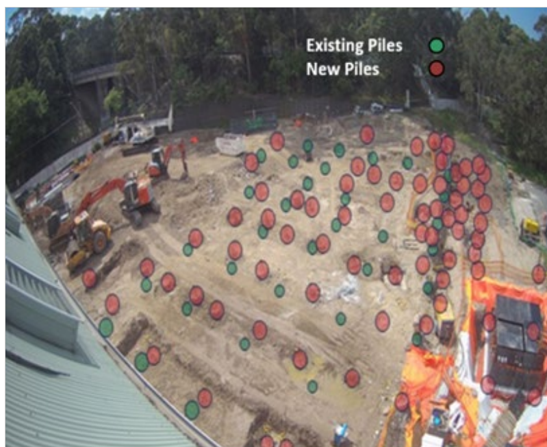
Figure 2 – Pile locations below old pool hall.
