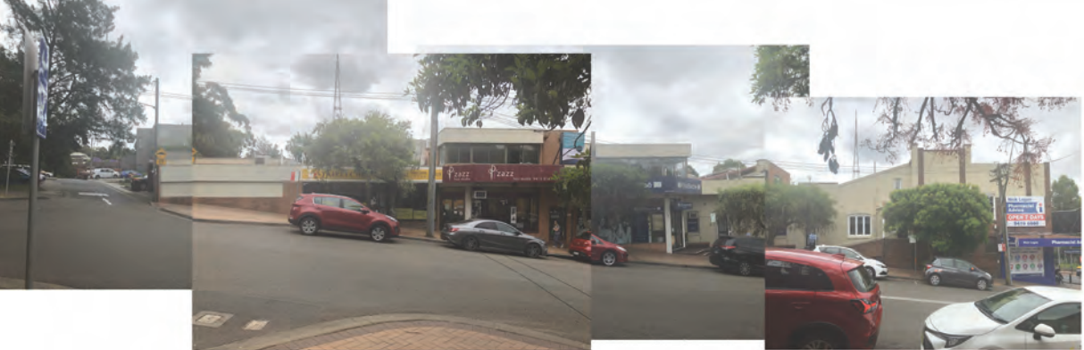
Fig. 2.17 | 2019 | Broughton Road looking North | Architectural Projects
