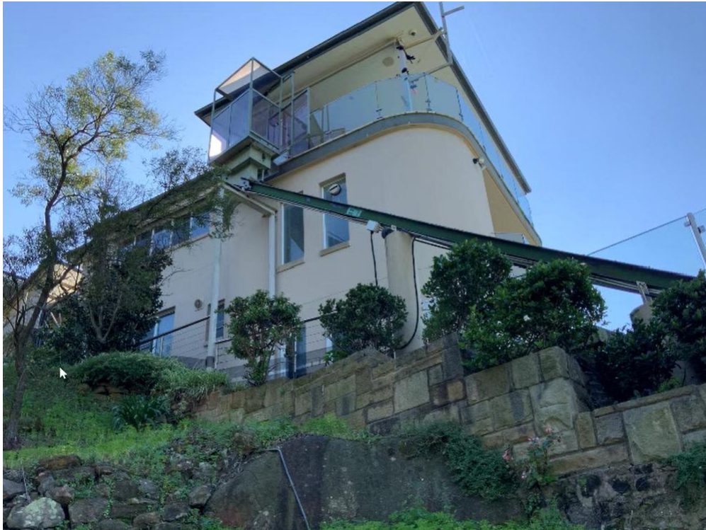
View of adjoining 3A Dorset Road from subject property – photo taken prior to demolition and approval of DA 2020/233; with DA 2022/105, currently under assessment, existing inclinator is proposed to be re-instated and re-furbished
