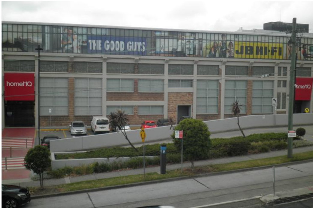
Figure 6: Western view of the subject building from Reserve Road
