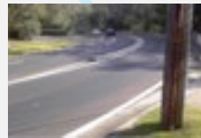
Road Pavements REPAIR Program
