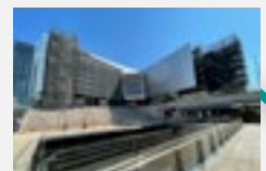
The Concourse cladding compliance upgrade
