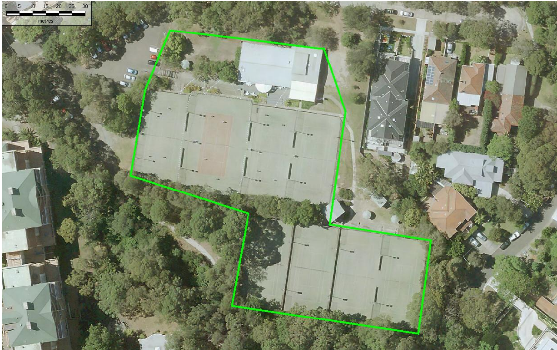
Talus Street Reserve – Talus Street, Naremburn
