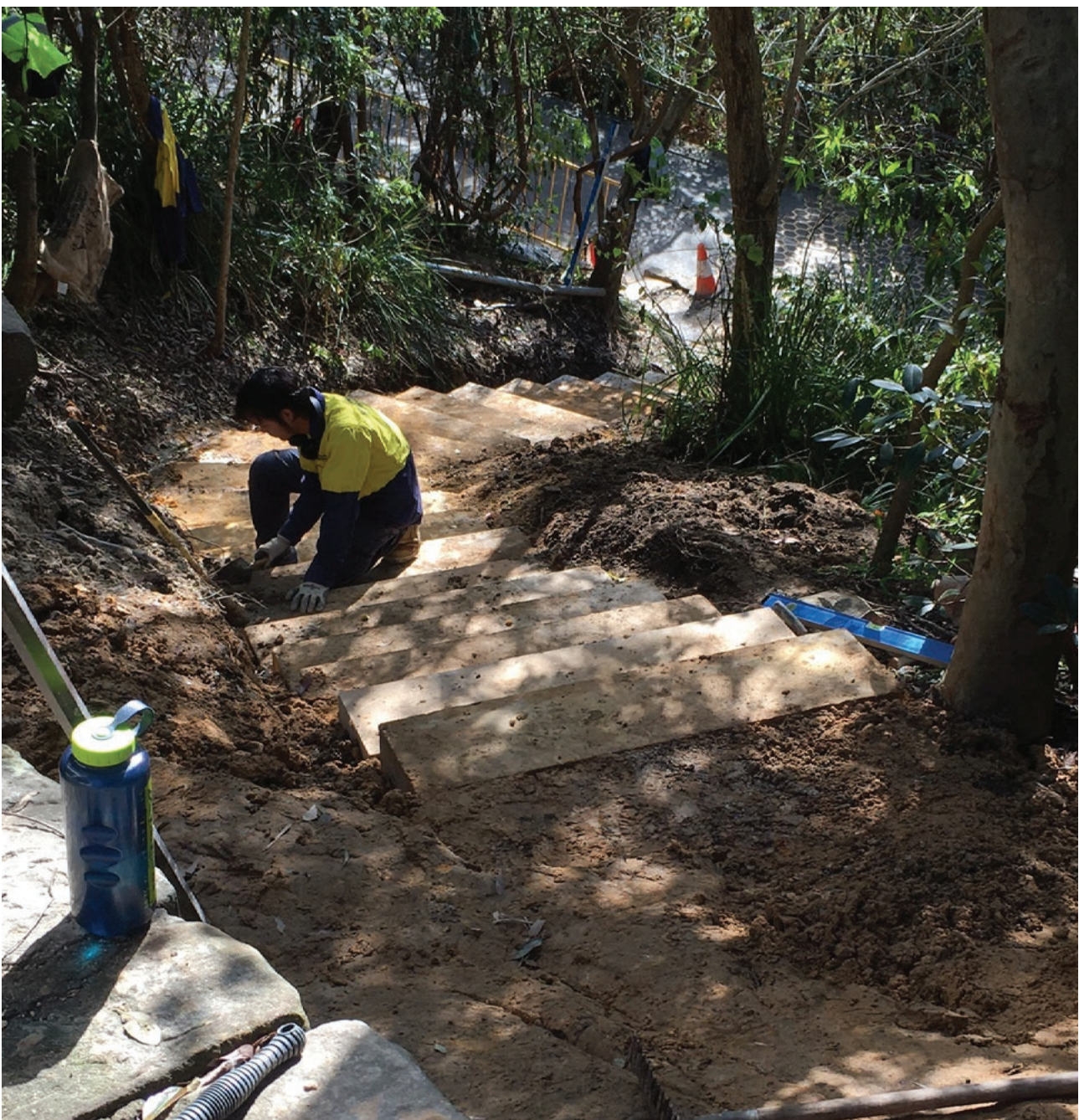
Replacement stairs being installed to improve access to Northbridge Baths
