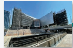
Completed cladding upgrade at The Concourse
