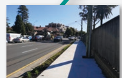
Construction commenced on shared cycleway
