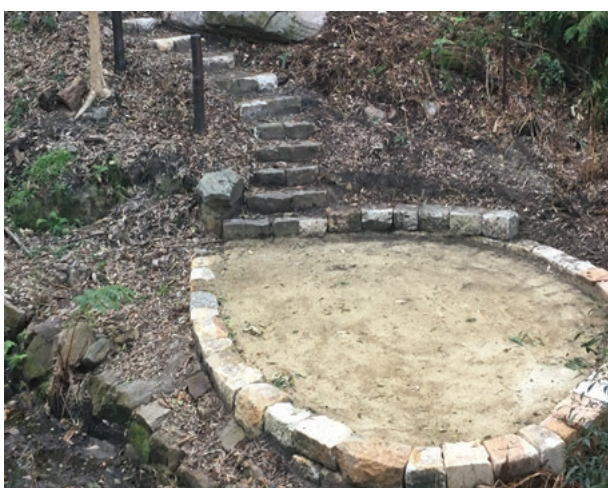
During 2021-22, the Haven Amphitheatre was upgraded
