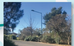
Northbridge Park car park lighting upgrade
