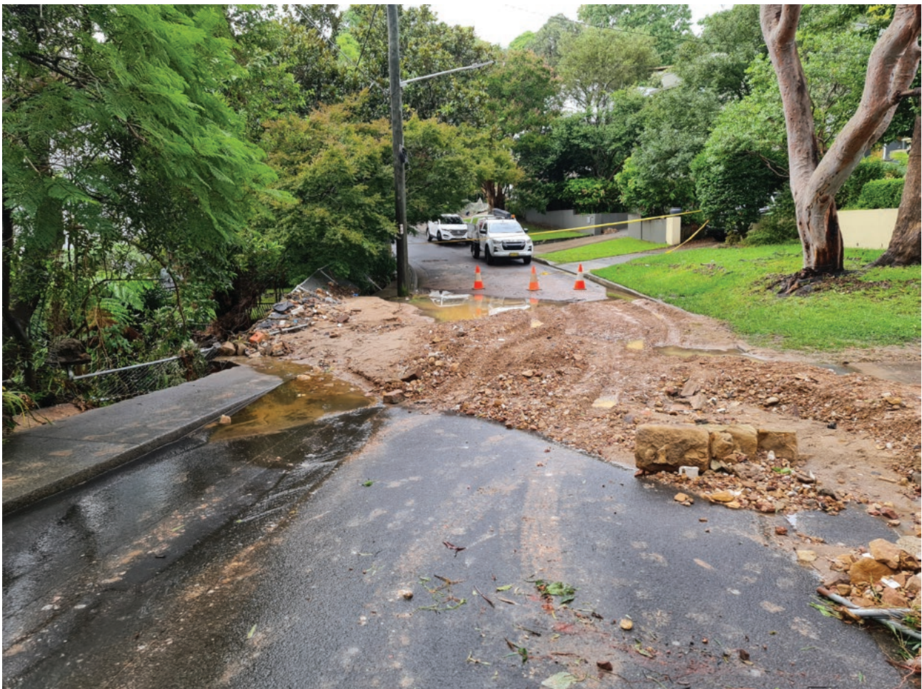
Impacts of flooding in Northbridge during March 2022
