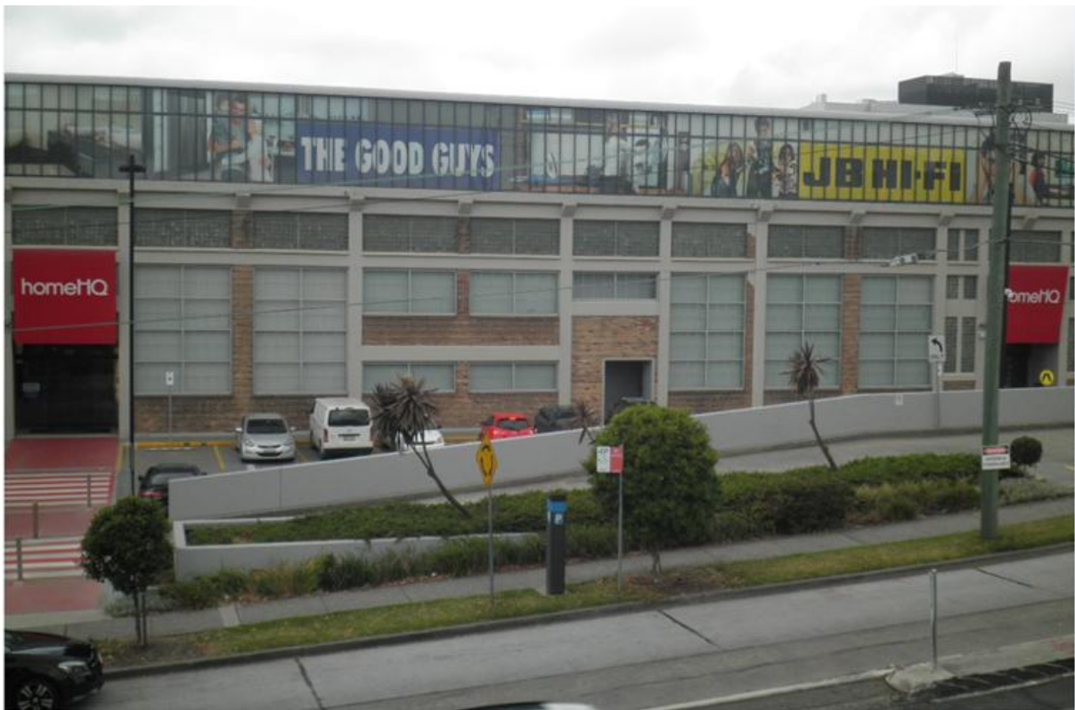
Figure 2: Western view of the subject building from Reserve Road
