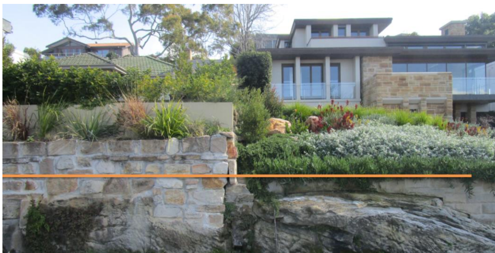
Current ground levels on Council's road reserve in front of 16 and 18 The Battlement
