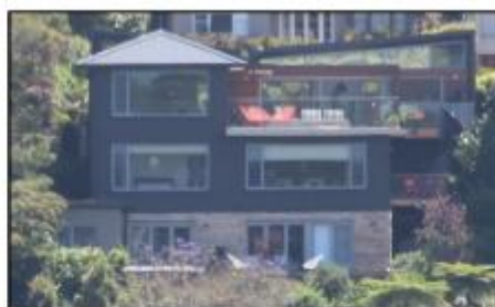
Photograph 5: No. 19 The Battlement, as viewed from Sailors Bay
