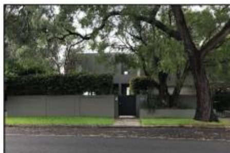
Photograph 7: No. 162 Edinburgh Road, as viewed from the street
