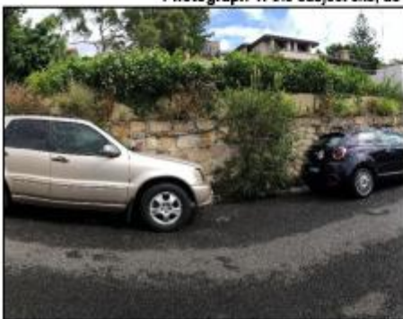
Photograph 2: The front retaining wall, as viewed from The Battlement
