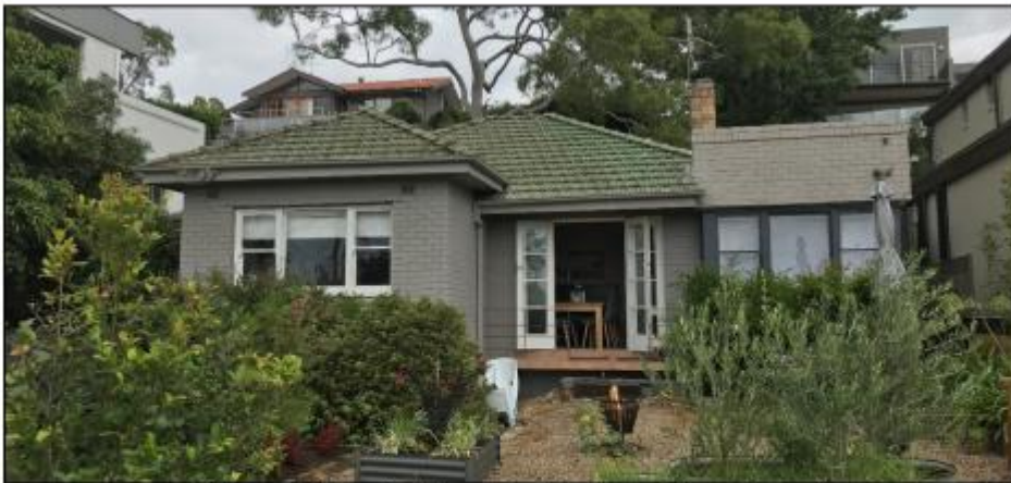
Photograph 1: the subject site, as viewed from the top of the retaining wall
