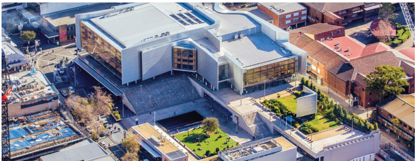
Figure 14: The Concourse, Chatswood
