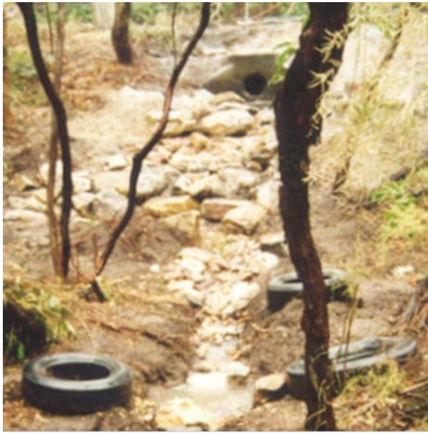
Figure 10 Rock-lined stormwater channel through bushland
