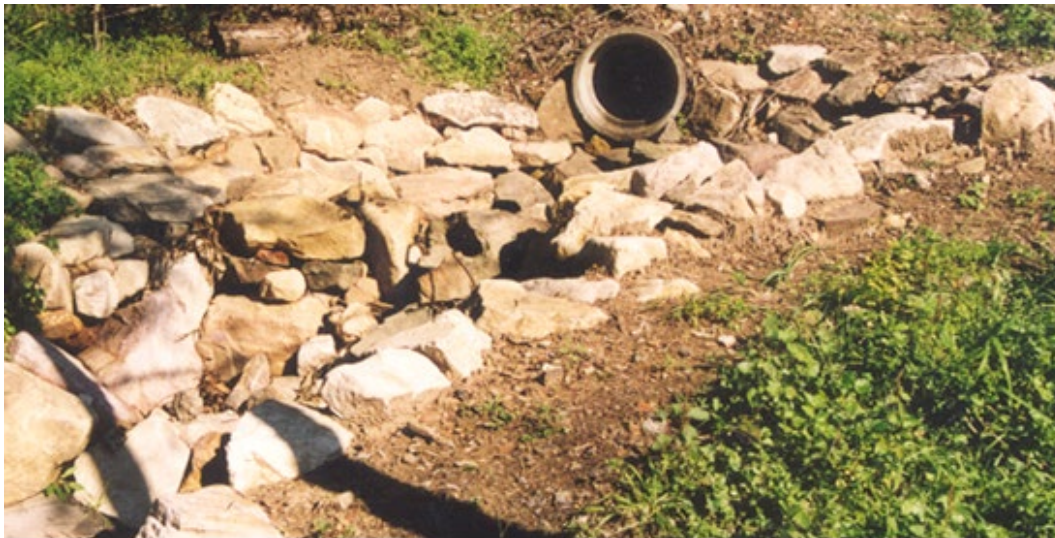
Figure 8 A rock lined channel from a stormwater pipe outlet
