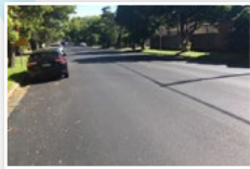
Archer St, Chatswood - renew road pavement
