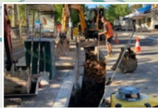
Willoughby Road and Merrenburn Avenue, Naremburn - stormwater upgrade
