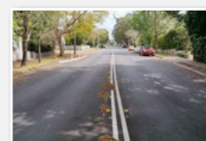
Smith Road to Clarendon Street, Artarmon - renew road pavement
