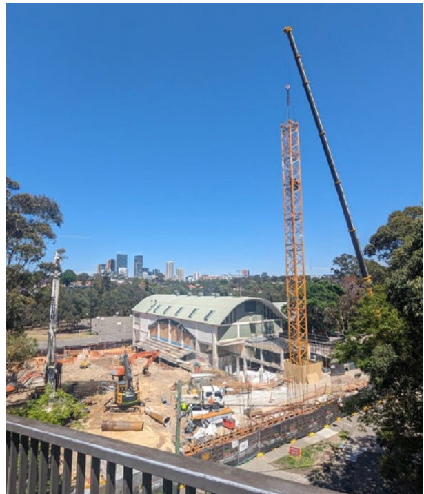
The tower crane is installed at Willoughby Leisure Centre.
