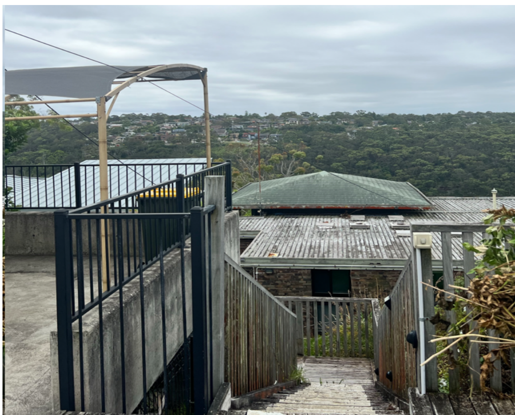
Figure 5 View of the existing house from the front boundary
