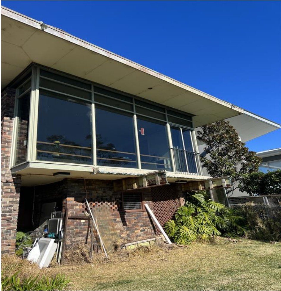
Figure 6 Rear view of existing house
