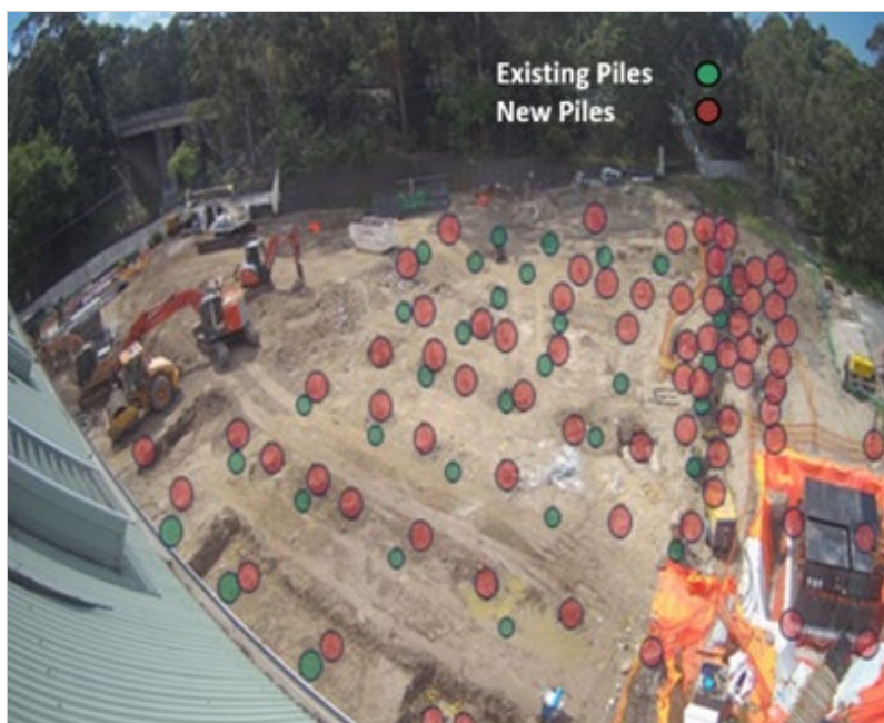
Figure 2 – Pile locations below old pool hall.
