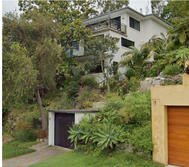
Figure 6: Front view of 57 Sugarloaf Crescent
