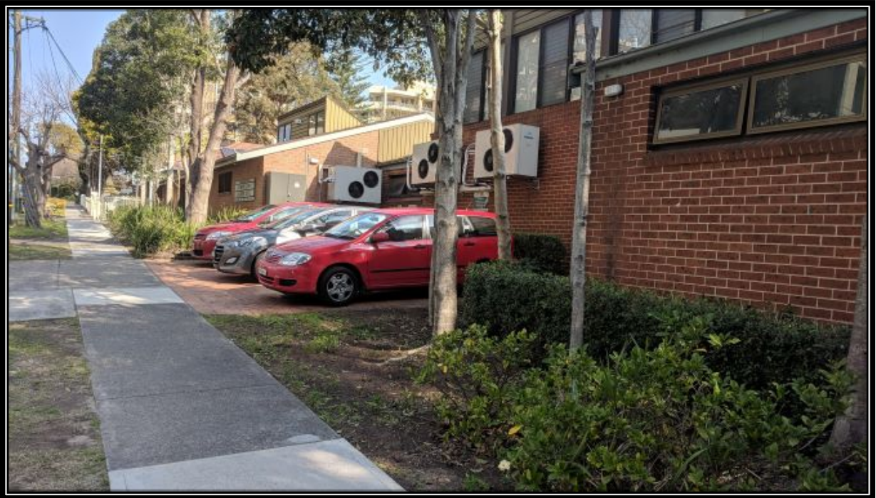
Photo 6 – 40 Devonshire Street from Devonshire Street frontage
