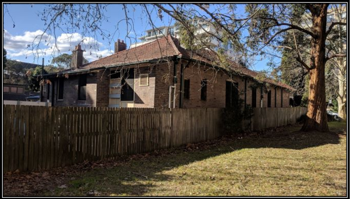
Photo 5 – Side of 28 Devonshire Street from Park Street
