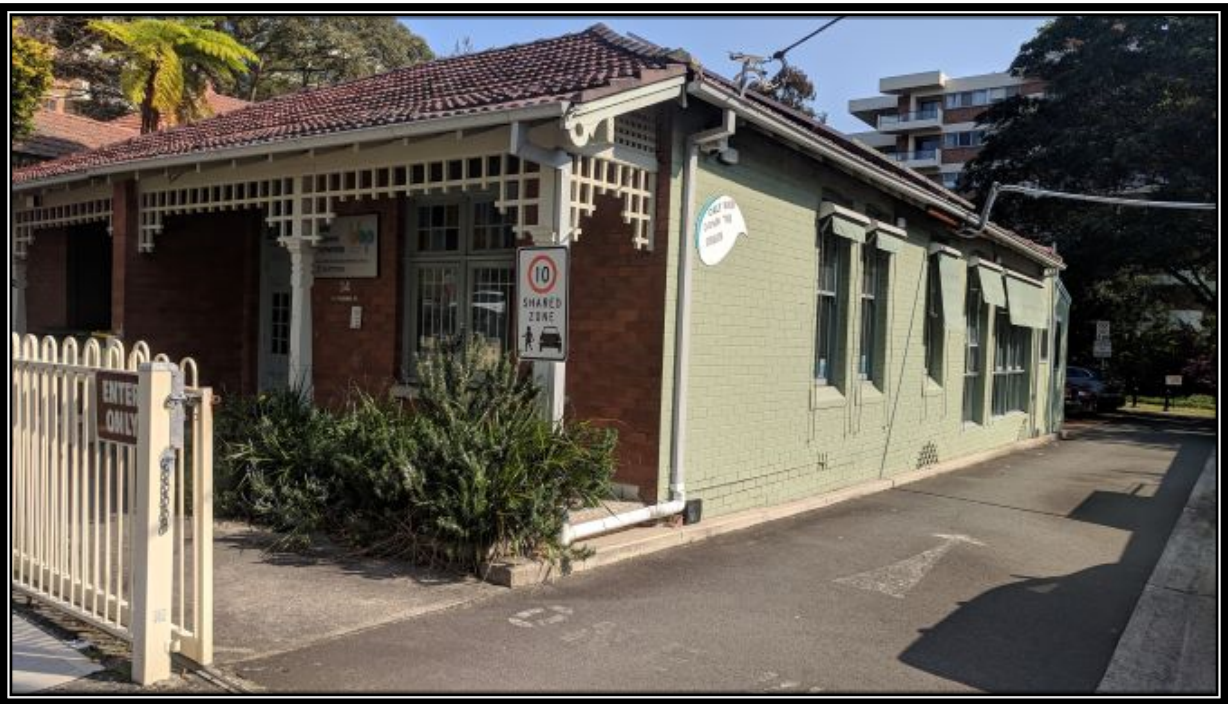
Photo 8 – 34 Devonshire Street from Devonshire Street frontage
