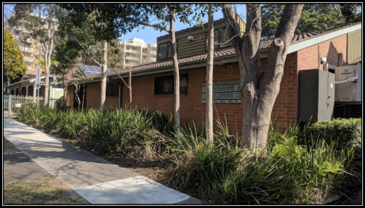
Photo 7 – 34 and 40 Devonshire Street from Devonshire Street frontage
