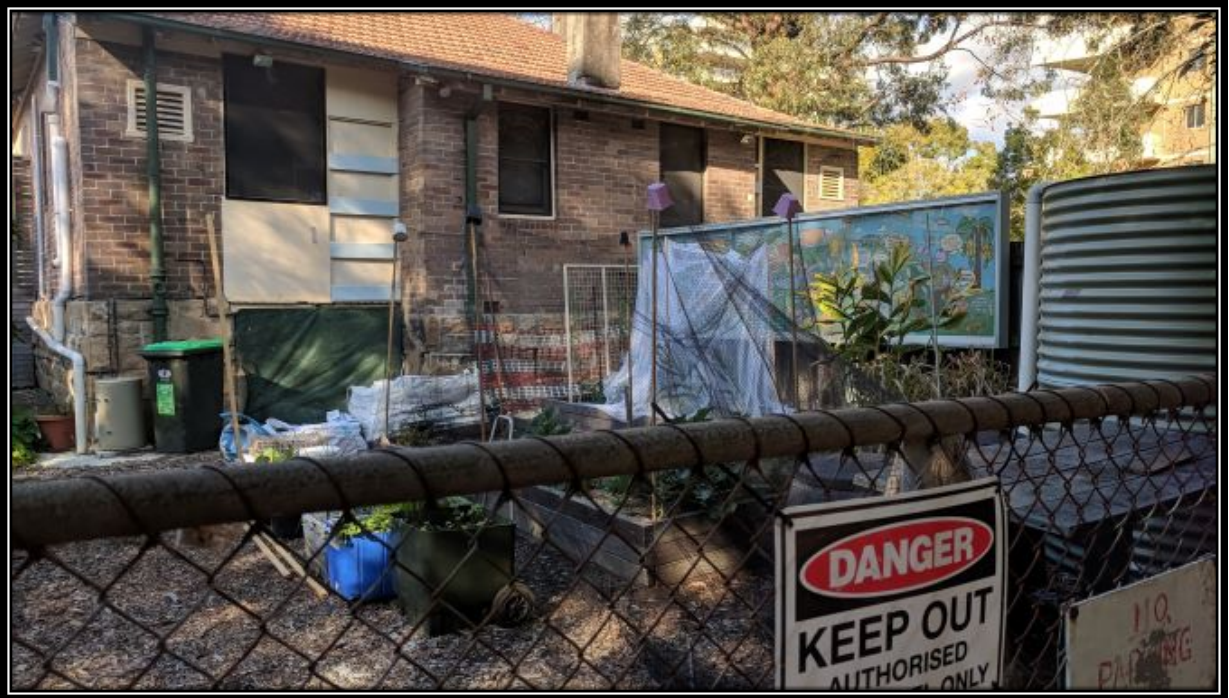
Photo 3 – Rear of 28-30 Devonshire Street.
